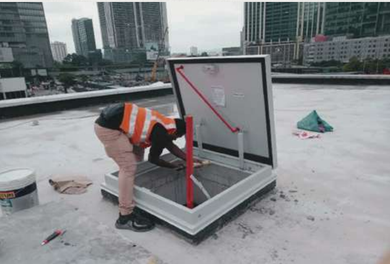
Roof hatch combined with attic ladder
