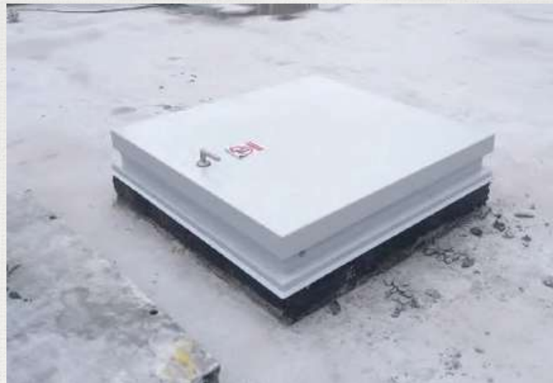
Roof hatch combined with attic ladder
