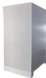
External Wall Ready Finished
