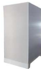
External Wall Ready Finished
